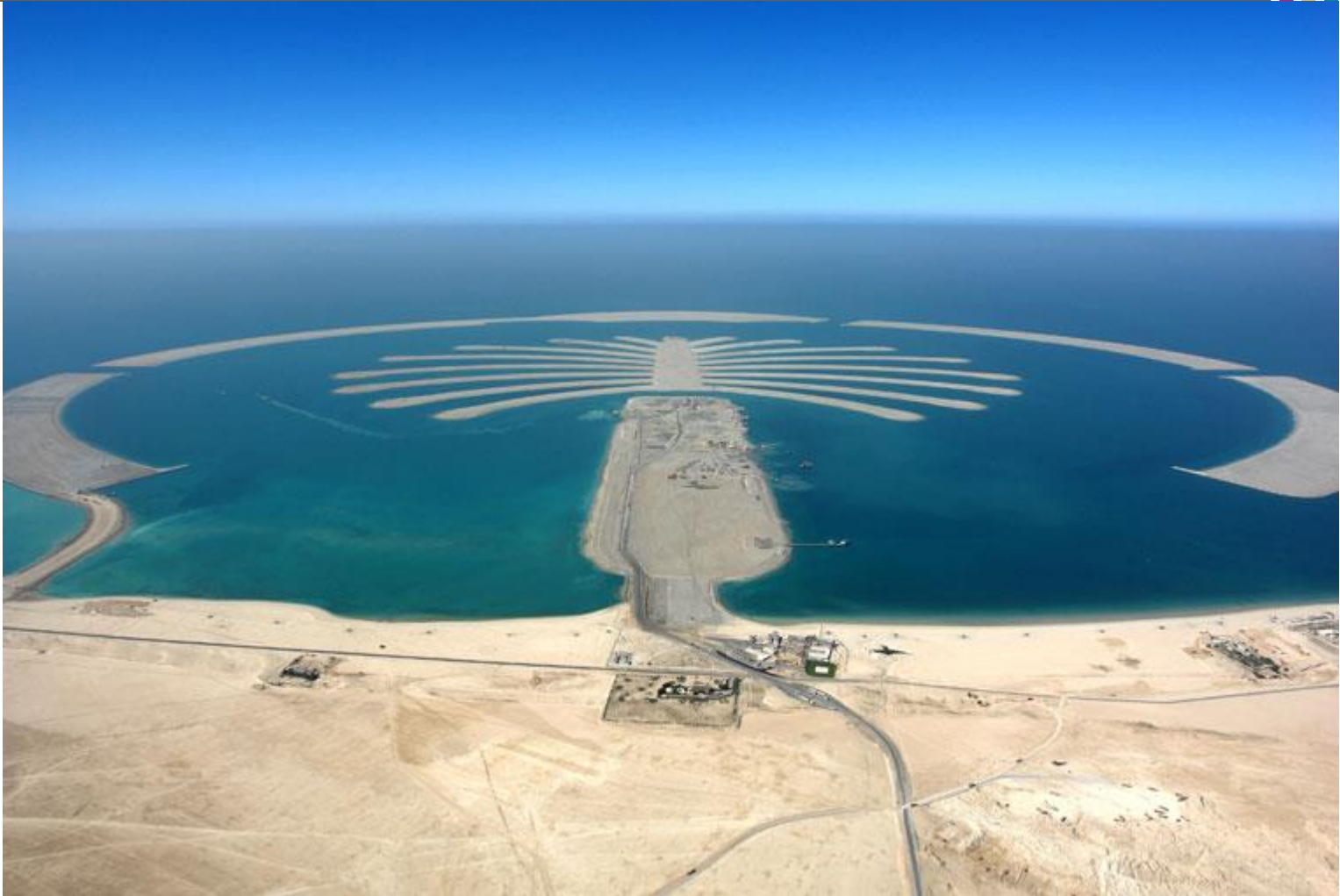
Dubai Palm Island II (Jebel Ali) - Dubai (U.A.E.) | 2004-2009 200,000,000 m 3 reclamation
