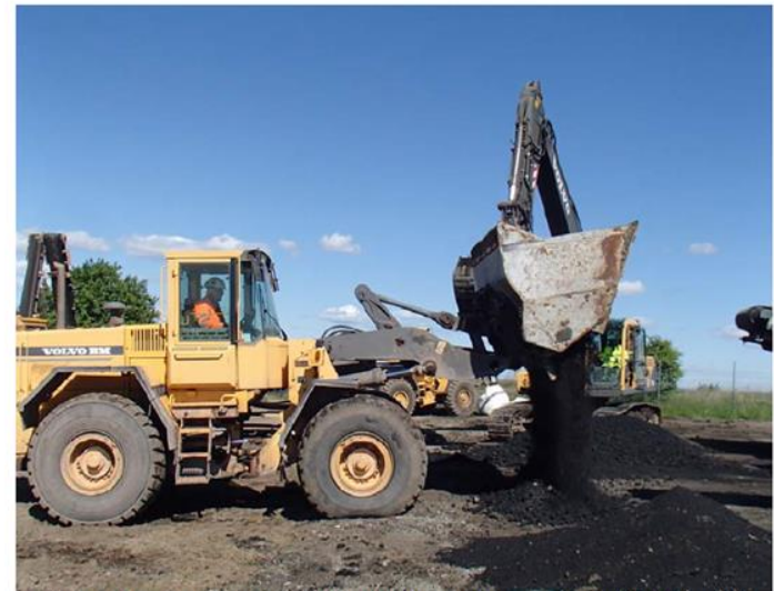
Picture 11 – Crushing of acid tar middle and oversize using ALLU bucket
